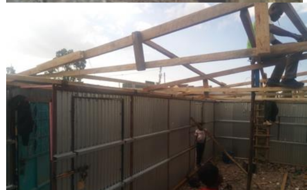
Above: the old office block Below: construction of the new classroom in progress
